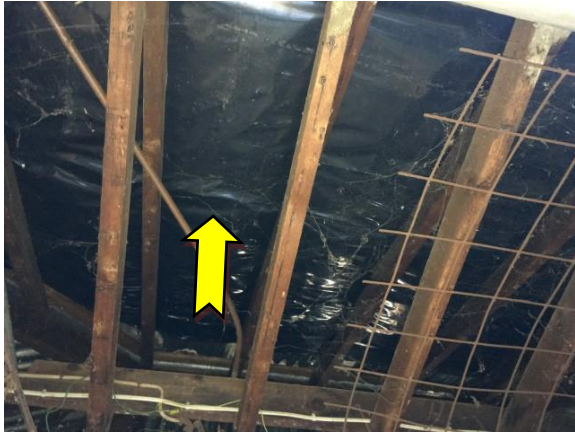
Photo 1. Interior, throughout, roof space – Suspected SMF sarking insulation.
